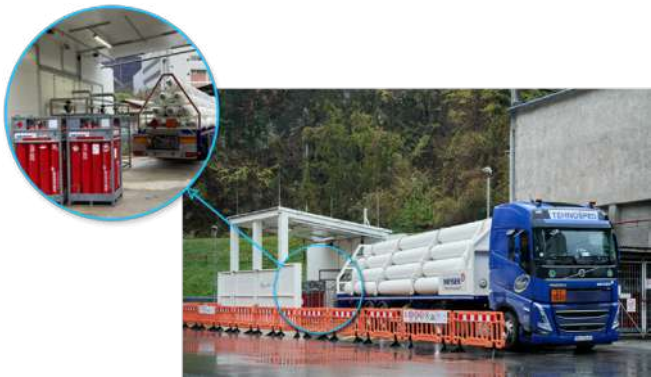
At Hrastnik1860, initial trials using trailer-supplied hydrogen have been successfully conducted, achieving a hydrogen intake rate of 60% in the oxyfuel glass furnace.
