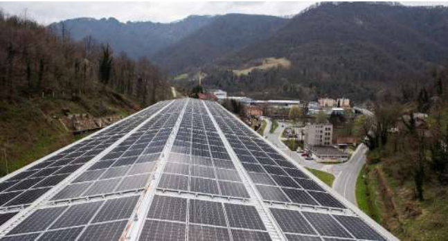
Rooftop photovoltaic system supporting the integration of renewable energy with the water electrolysis system and glass furnace.
